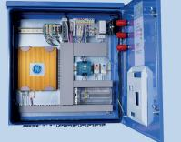
A modular and configurable system that can monitor the various key components of a power transformer listed here, depending on the asset owner's requirements.
